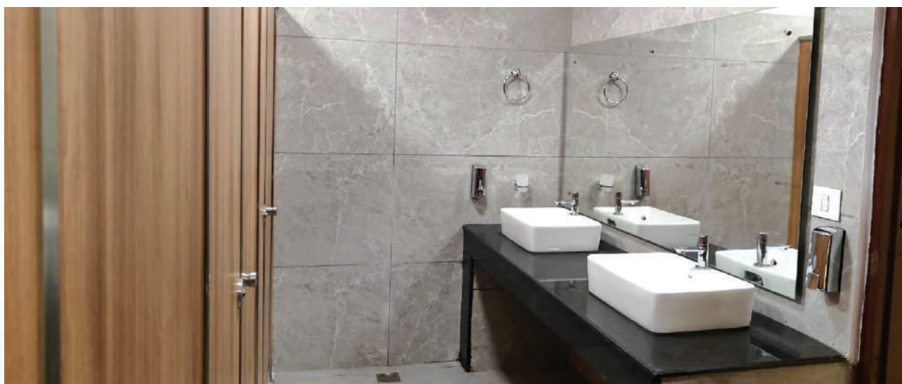
Renovation of Rest Rooms at Prashant Sadan
