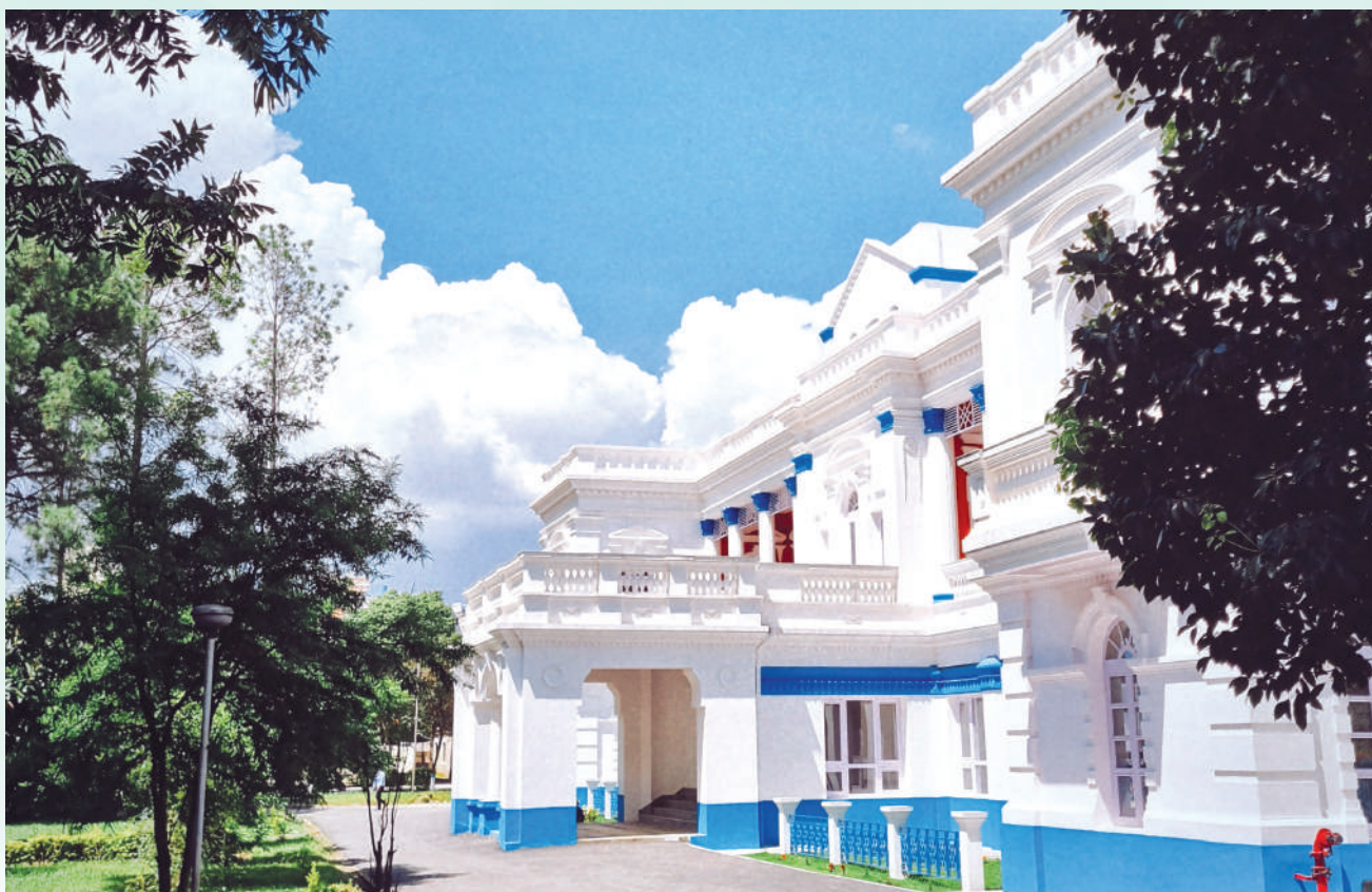
Sampada Sadan as viewed from the Southern side
